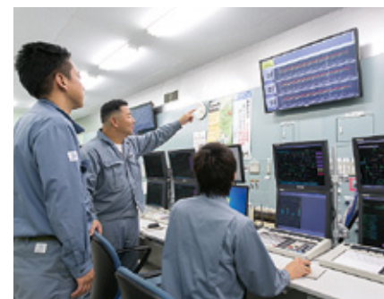
Instrument panel room for monitoring the entire operation of the anone manufacturing plant. The large 65-inch monitor is installed above the APS5000 monitoring/control panel. The monitor displays the APS5000's monitoring screen during normal operation. When an alarm is generated, the display automatically changes to the ACTMoS's monitoring screen. All members present in the room can grasp the condition of the generated abnormality so that they can conduct response activities in cooperation.
