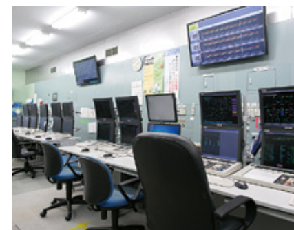
General instrument panel room where the operation of two anone manufacturing plants is monitored and controlled.
