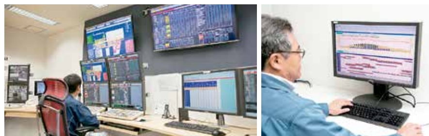
Left: The central monitoring room at the Ariake Minami plant. Operators at the three plants can now share the same view through their screens in their central monitoring rooms, which enables them to reference information about problems that occurred at other plants and how they were handled. The current operation support system has implemented a unique function that shows the approximate price in yen of the electricity and/or gas being used to produce one gigajoule of energy. Right: The same operation support system monitors can also be accessed and viewed from offices at the headquarters, allowing relevant departments and management personnel to check the status of operations.
