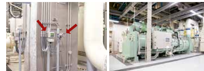
Left: A MagneW™3000 FLEX+ electromagnetic flowmeter measures flow rate while a DSTJ3000 Ace+ transmitter measures pressure. Right: A turbo chiller uses electricity to produce chilled water.
