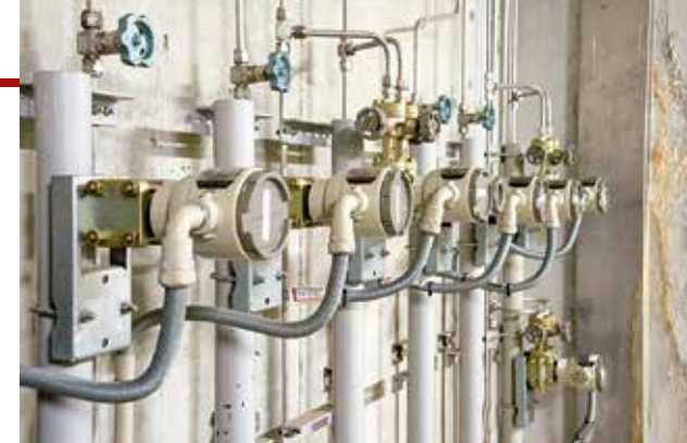
DSTJ™3000 Ace+ differential pressure transmitters measure the pressure of the main pipes for heat and chilled water.
