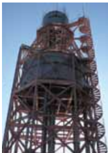
Elevated water tank for flow calibration rig
