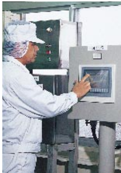
A Takara Shoyu Co., Ltd., employee uses an EST330 operation display to monitor the liquid mixing process for dip sauces that exploit the savory flavor of soy sauce at the company's Choshi Plant.
