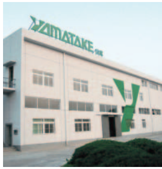
Nanqiao Factory A configuration factory that started operations in November 2003.
