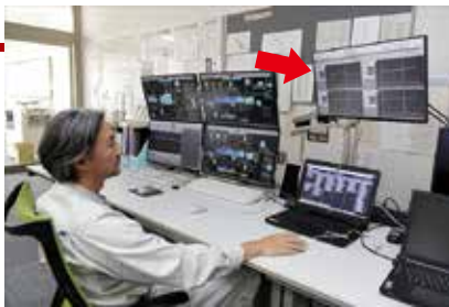
The Advanced Critical Trend Monitoring for Safety system running at the Water Purification Management Center can be linked with other companies' monitoring systems. It can make predictions with only one analog data collection input point, without the need for complicated conditional settings, which is an advantage of the system.
