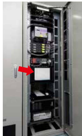
Azbil's Plant Information Management System, which has been operating as a data management system since before the introduction of Advanced Critical Trend Monitoring for Safety. It centrally stores and manages operating data from various facilities, including data collected by other companies' monitoring systems. It is used for monitoring and analysis of operating conditions.
