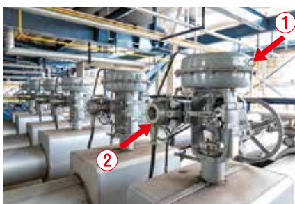
① Pressure-balanced cage type control valve equipped with ② 700 Series Smart Valve Positioner. The valve controls the flow rate of steam that is supplied with the raw materials for petrochemical products.
