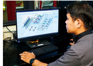
A savic-net™G5 monitoring screen for the new BEMS. The operating status of equipment can be checked with easy-to-understand graphics.
