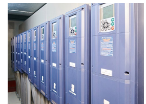
Pumps (left) send chilled water and cooling water to the air conditioners while VSDs (above) control the variable flow rate of the pumps.
