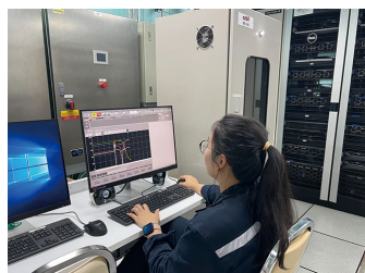
An engineer uses Azbil’s control performance optimization design tool in the control room to check the operational data collected from the existing DCS.
