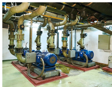
Pumps (left) send chilled water and cooling water to the air conditioners while VSDs (above) control the variable flow rate of the pumps.
