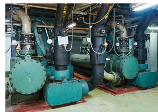
Chillers in the heat source machine room produce chilled water for air conditioning. The BEMS automates the start/stop of equipment according to schedules and controls the number of units that are operating.
