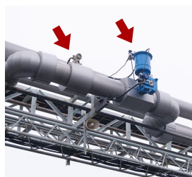
Eccentric rotary control valve FloWing™ for controlling the pressure of steam immediately after it is sent out of the boiler (right) and steam flowmeter STEAMcube™ (left).
