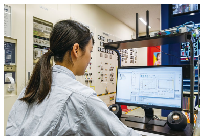
On the Valstaff screen, the stick-slip *5 diagnostic parameters of the main steam temperature control valve can be checked in a graph
