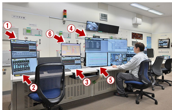
Monitor screens for the DCS Harmonas-DEO (①, ②, ③, ④), SORTiA-MPC (⑤), and Knowledge Power (⑥) installed in the central monitoring room.
