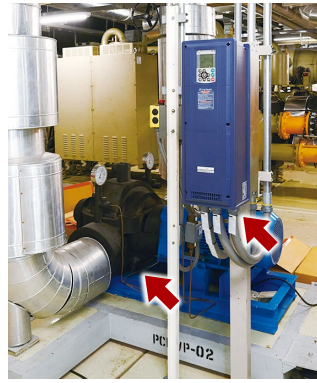
A primary chilled water pump for HVAC equipment (left) and an inverter that controls the pump's rotation speed according to demand (right)
