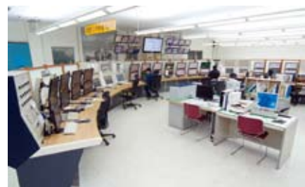
The Advanced-PS APS5000 system is circularly arranged in the instrument panel room. All monitors are visible from the center of the room to allow easy confirmation of equipment operating status by the supervisor.
