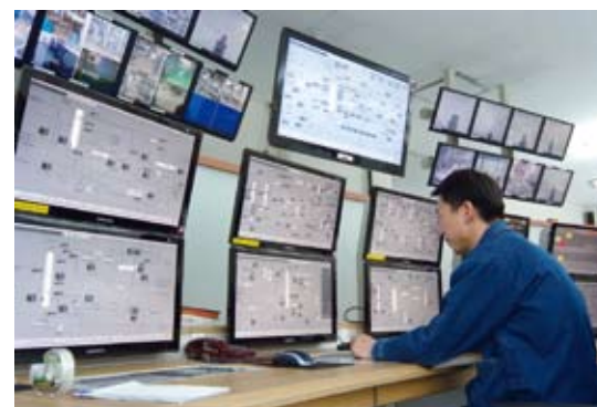
For the monitoring and control screens, the IOUS 500 Windows-based human-machine interface is used. The well-designed display layout, including a large LCD display and sets of two display panels arranged vertically, has expanded the monitoring and control range for each operator and increased dramatically the amount of displayed information.
