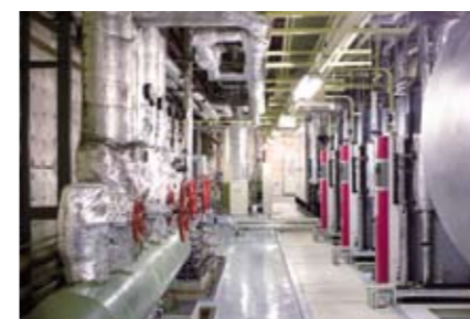
Machine room installed with highly efficient once-through boilers and cogeneration system as part of the project. Many visitors come to see this system.
