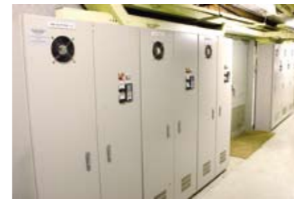
Yamatake-manufactured inverter control panels installed in the machine room. They optimize energy consumption by providing appropriate control according to the air-handling units and pump load demand.
