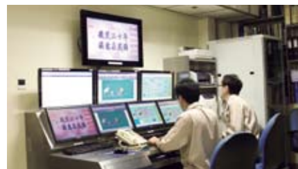
The savic-net FX installed as part of the project and existing monitoring system. The savic-net FX installed as a BEMS links with the existing system for monitoring, managing and analyzing the energy consumption trends.
