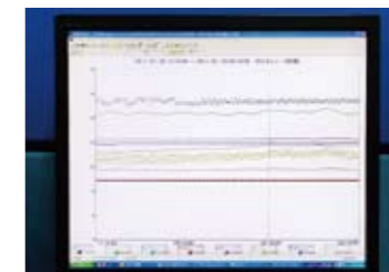
Screen on the client terminal of the PREXION installed in the office. This terminal displays the history and trend data of the production facilities' operating status, which are used to investigate the cause should a problem occur. MELS installed the PREXION in Plant No. 1 and also decided to install it in Plant No. 2. This tool is also utilized in making process improvements.
