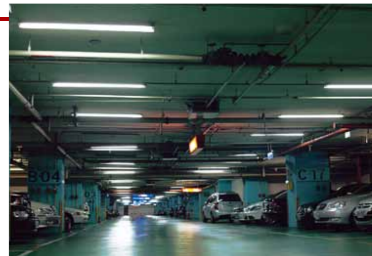
Parking area lights were replaced with energy-efficient ballast-equipped lighting.
