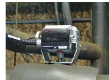
ACTIVAL PLUS Motorized Two-Way Valve installed on a chilled water coil piping for HVAC. An all-in-one valve with the functions of a control valve, flowmeter, pressure gauge, and thermometer, a significant cost saving is possible when these functions are used together.
