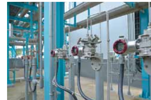
The SuperAce™ AT9000 Advanced Transmitter for pressure and differential pressure is used in the air separation process of gas production.
