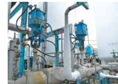
HTS top-guided single-seated control valves can endure the low temperatures of the air separation process. Equipment that controls liquefied oxygen at -190°C must have high durability at super-low temperatures. Due to the ultralow temperature liquid, part of the piping is covered with frost.
