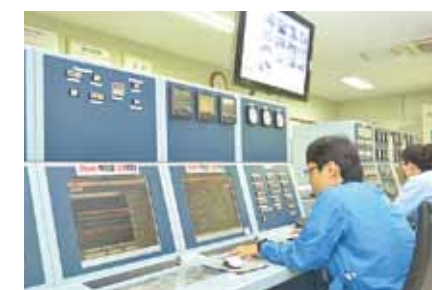
Harmonas-DEO control and monitoring terminals in the central monitoring room. The system enables a minimum of only three regular operators to monitor both the first and second plants at Ulsan.
