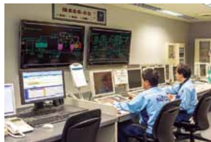
The monitoring room of the airport's central heating and cooling plant, where Advanced-PS and the utility optimization software package are installed.
