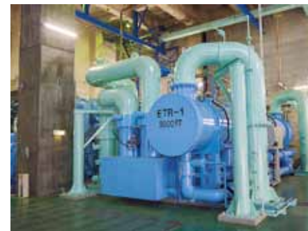
An electric chiller in the central heating and cooling plant.
