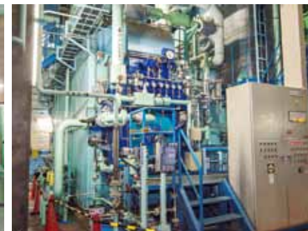
A two-drum water tube steam boiler.
