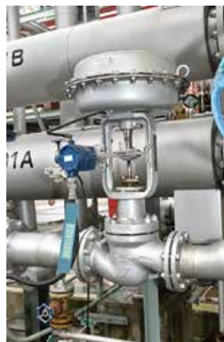
A smart valve positioner and single-seated control valve operating in a styrene monomer production facility. Data on valve operation is sent from the positioner to the maintenance support system so that warning signs of a problem can be detected quickly.
