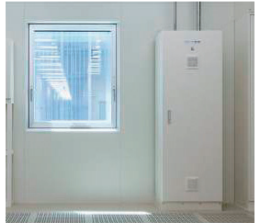
Fig. 5. Window in a cleanroom
