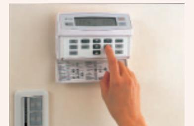
A controller for humidity, temperature and ventilation
