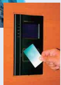
The security system is made up of savic-net ssEV, a monitoring system designed solely for security purposes, card readers compatible with contactless IC cards and a management system for the key-hold box compatible with these cards. This is a large-scale system comprising some 90 card reader controllers and around 700 contactless IC card readers for the roughly 20,000 cards issued to building users.
