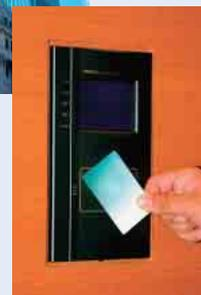
The security system is made up of savic-net ssEV, a monitoring system designed solely for security purposes, card readers compatible with contactless IC cards and a management system for the key-hold box compatible with these cards. This is a large-scale system comprising some 90 card reader controllers and around 700 contactless IC card readers for the roughly 20,000 cards issued to building users.
