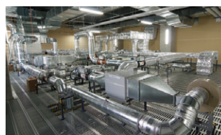
Clean room air-conditioning experiment facility in the advanced technology laboratory building
