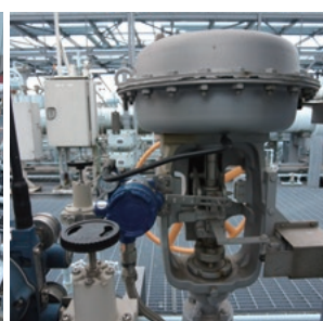
The HIBIKI LNG site and Azbil's smart valve positioner comprising the control valve maintenance support system
