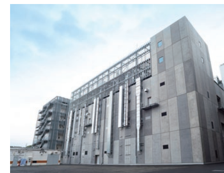
Building 104 · Center for developing measurement and control technologies with expanded facilities for MEMS sensor development and production using world-class MEMS technology · Enhanced facilities for developing measurement standardization technology, which is the basis for high-precision, high-reliability products
