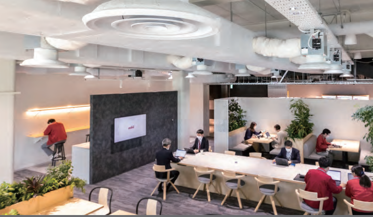
• 1st floor café-style workspace of Building 103 A skeleton ceiling allows plumbing and equipment to be seen
