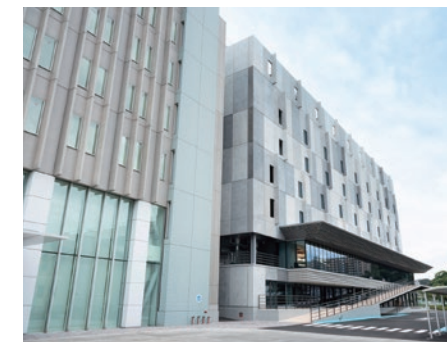
Building 103 · Featuring improved facilities for the development of central air-conditioning technology that offers superior comfort, energy efficiency, and harmony with the environment · An innovative development environment that stimulates and activates creativity
