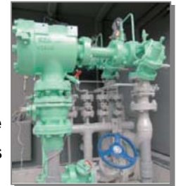
▼ Pressure regulator (MAFV governor unit)
