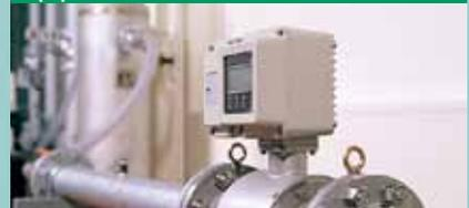
This product offers high response of 160ms scanning speed which makes it appropriate for a variety of high-speed equipment. Its high rangeability covers a wide range of flow measurement, thus eliminating the use of multiple meters.
