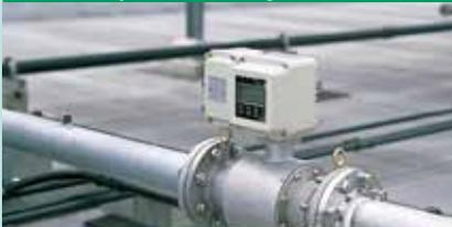
A mass flow meter is necessary to measure the actual load and air consumption of a compressor. This product can precisely measure the flow with no need for adjustment in temperature and pressure.
