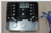
Remove wiring from Q270A.
